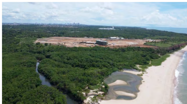
Figure 5. Tauá Resort construction
