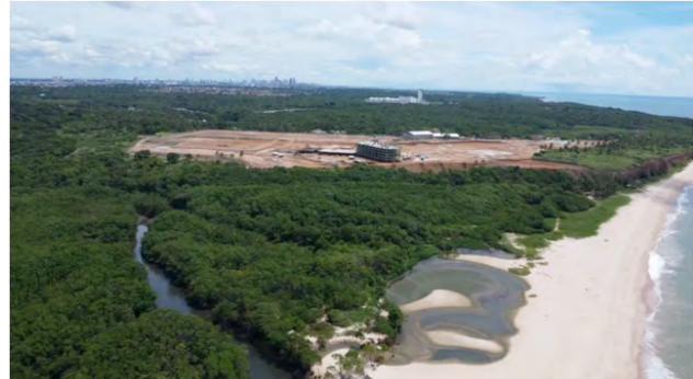
Figure 5. Tauá Resort construction
